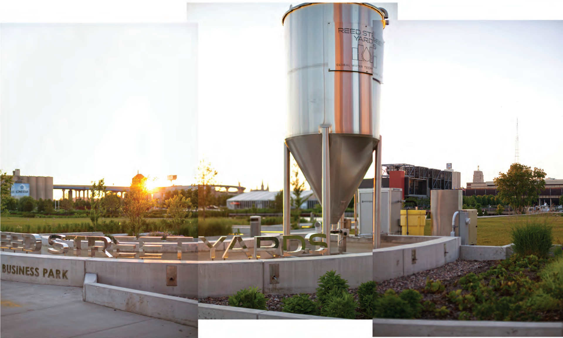
Reed StreetYards eco-industrial zone, Milwaukee
