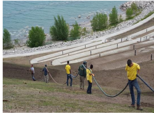
The Biotic Earth Black, native seed mix, tackifier, and fertilizer was applied hydraulically.
