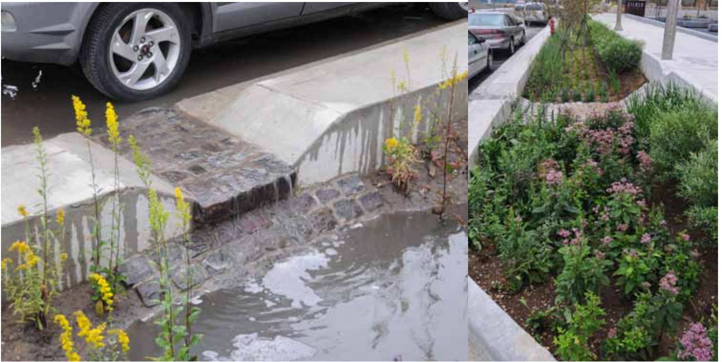
Pabst Brewery Redevelopment, Rain Garden Bioswale
