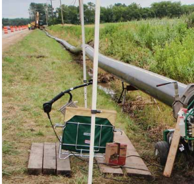
MMSD's Landfill Gas Pipeline Project
