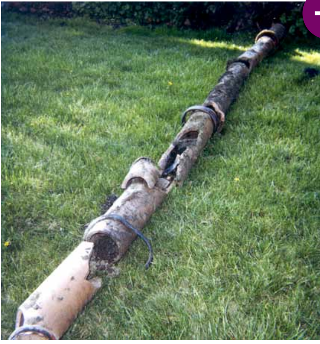
Leaky Lateral Pipe
