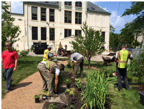
▲ The most recent phase at Maryland Avenue Montessori includes a bioswale that captures water from the school's roof, a new walking path, trees, and perennial plants. The school plans to create plant identification tags for student and community use in a future phase. New plantings mimic nature, providing a mini wildlife sanctuary with birds, rabbits, and insects for the dense neighborhood.
