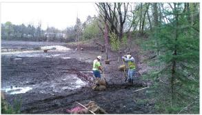
material, additional shoreline stabilization efforts were completed through the installation of thousands of live stakes and other plant material on shoreline slopes including hundreds of container shrubs. Cardno also installed 200+ large ball and burlap trees throughout City of Cedarburg Parks and multiple
