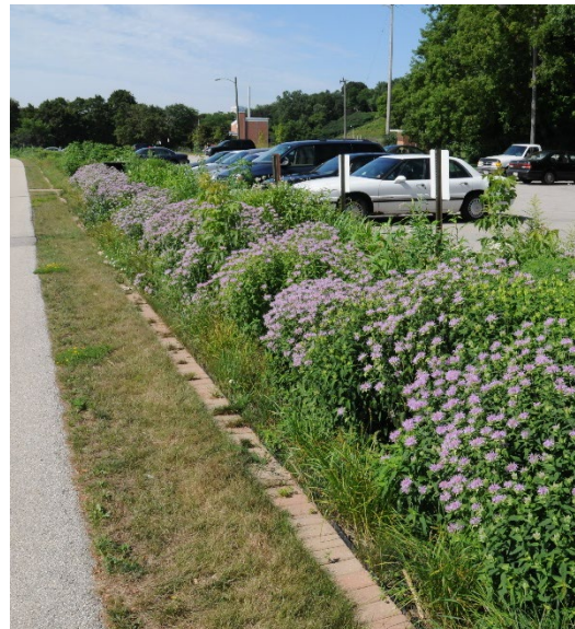
Bioretention areas not only attenuate stormwater that would otherwise drain directly to streams, but also provide habitat for birds, bees, and native vegetation; improve water and air quality; reduce street noise; and may improve the health of local residents. Photo credit: MMSD
