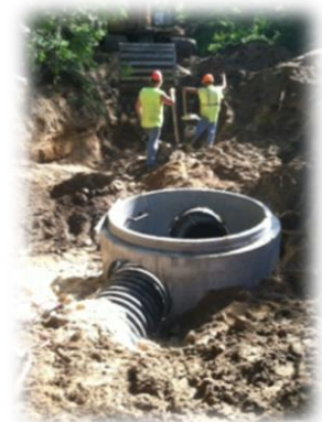
Installation of stormwater BMPs
