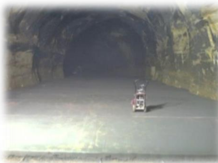
Newly installed road inside the mine portal
